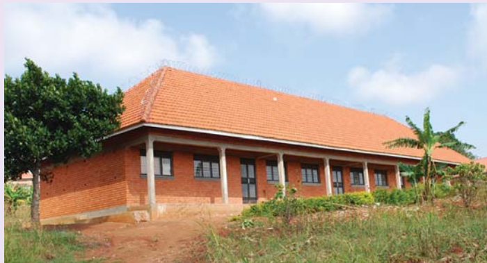
The school's classroom building is complete. Work remains to be done on the dormitory and dispensary, restrooms, and office buildings
