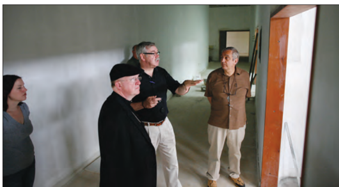
During a tour of the hospital, Peter Flynn, diocesan director of Finance and Administrative Services, talks about one of the operating rooms with Bishop Vann (center) and St. Elizabeth Ann Seton parishioners Alan Napleton (right) and Kirstin Kloesel (left).
