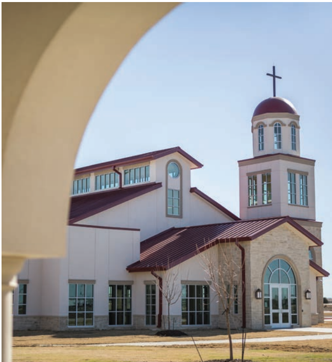
Part of a $17-million masterplan, the St. Martin de Porres Parish Hall is adjacent to the new St. Martin de Porres Catholic School dedicated Nov. 3, 2017. A church and gymnasium are future projects. (NTC photo/Juan Guajardo)
