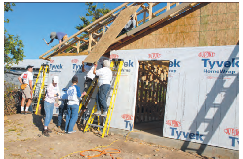
Volunteers work to build the house in the Fall.
