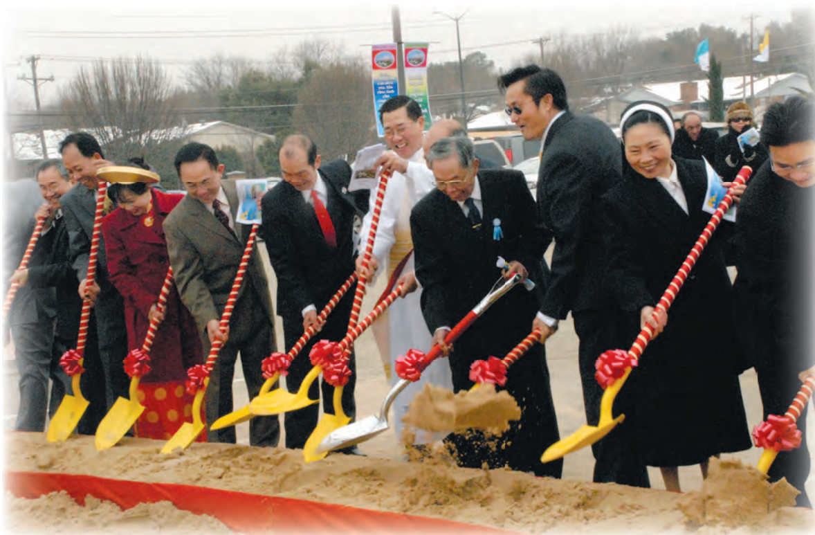
Several parish benefactors and clergy turn the first shovelfuls of dirt during the groundbreaking. Said Fr. Polycarp, pastor at Vietnamese Martyrs, "God was working with us to build a place where we can worship and glorify Him."
