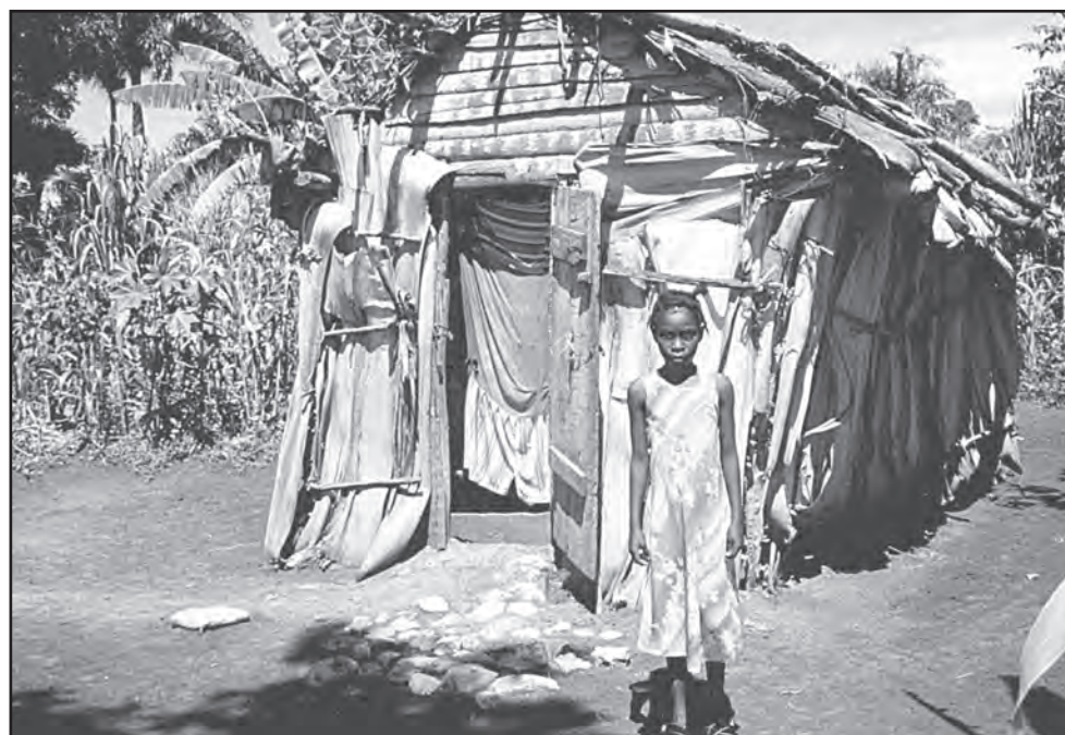
Typical housing in Haiti’s Central Plateau — a leaky patchwork of canvas, old plastic and scraps of wood.
