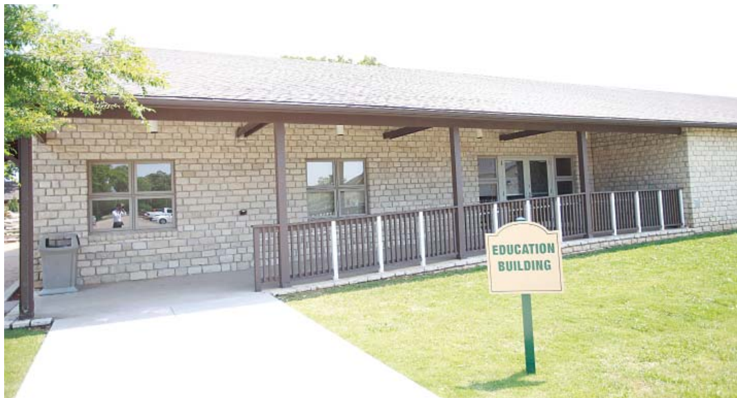
The Education Building classrooms at the parish were converted into apartment-style housing for families who lost their homes in the tornado. Many of those families are expected to continue living there until September which is when most of the houses are expected to be repaired.
