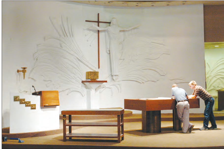
Dan Voelkel, left, and Rob Mittelbronn of Norman Voelkel Construction look over blueprints for the renovation of St. Clement of Rome Church in Metairie, Louisiana, July 25. After the church sustained extensive flood damage from Hurricane Katrina, the parish relocated Masses to an adjacent gymnasium. The parish plans to reopen the church for Mass in August. (CNS photo/Mike Crupi, CATHOLIC COURIER)
