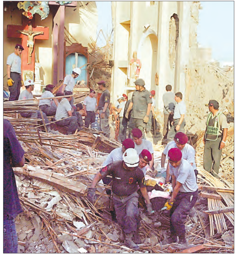
RESCUE EFFORTS — Rescue personnel work at a destroyed church in Pisco, Peru, Aug. 16, after a major earthquake struck the evening before, killing hundreds of people, mainly south of Lima. (CNS photo/Mariana Bazo, Reuters)
