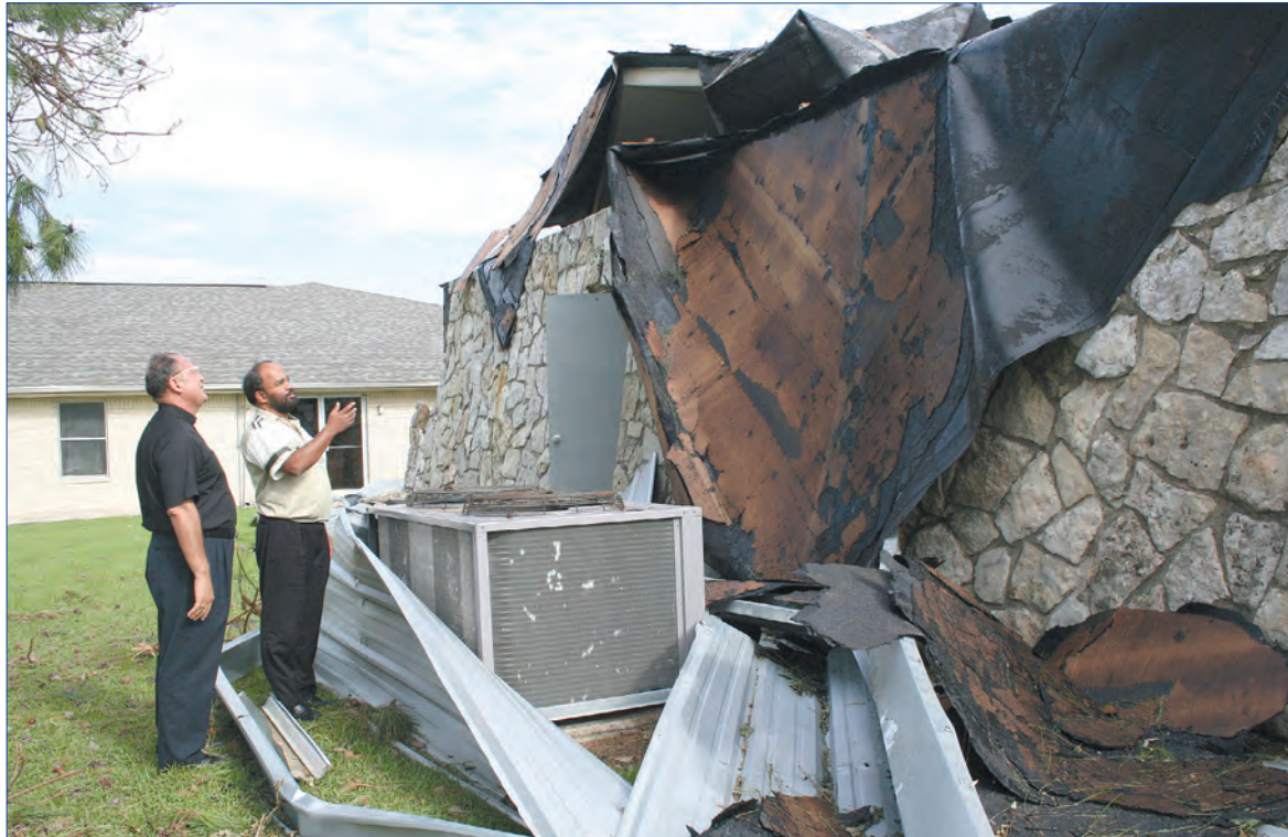
Carmelite Father Joseph Kattakkara, pastor of St. Mary Church in Fannett, shows Beaumont Bishop Curtis Guillory, Sept. 16, where the roof was ripped off the church by Hurricane Ike. When the storm hit Sept. 13, the entire roof was torn off by the 100 mph winds, leaving only the plywood decking. (CNS photo/Sarah Dupre, EAST TEXAS CATHOLIC)
