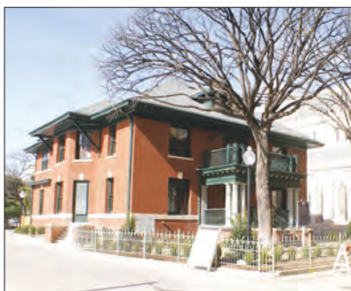
The rectory renovation project was completed in the spring of 2009. (Photo courtesy of OA&ID)
