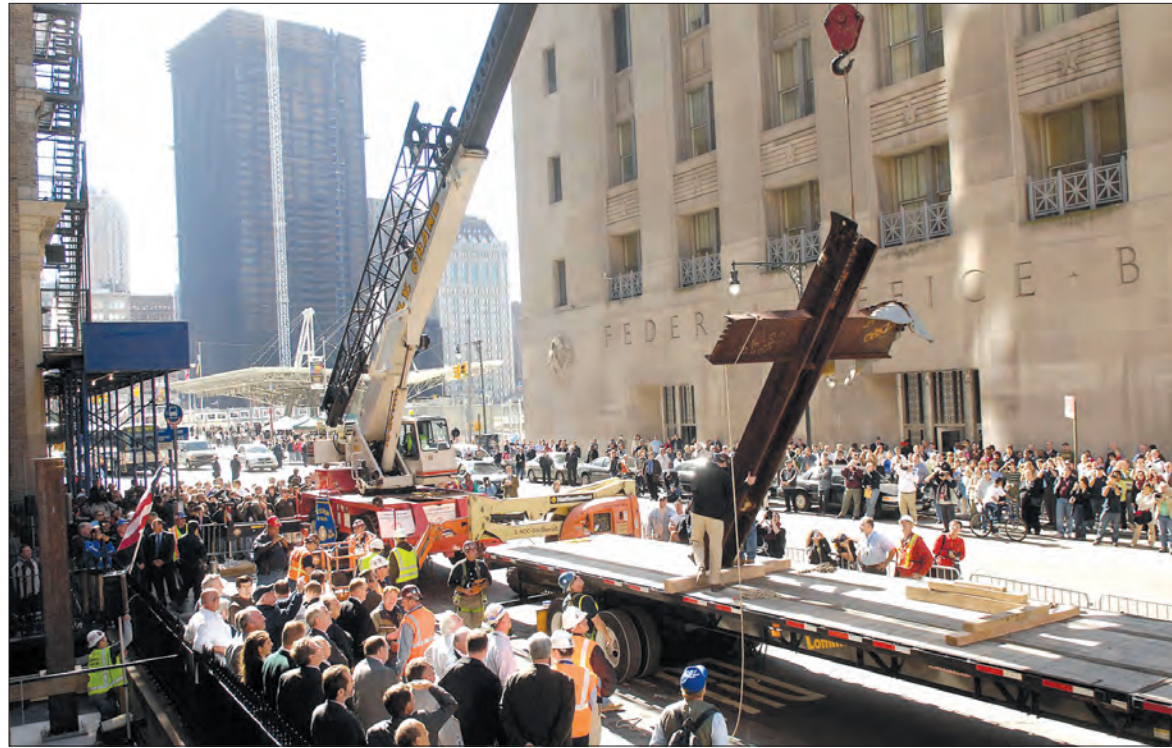
CROSS MOVED — Construction workers Oct. 5 remove the 20-foot cross formed by steel beams that was recovered from the rubble after the Sept. 11, 2001, attacks brought down the World Trade Center in New York. The cross was taken to nearby St. Peter's Church, where it will be stored as reconstruction on the trade center site continues (CNS photo/Chip East, Reuters)
