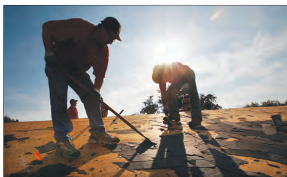
Jim Kinser (left) and Michael Sommerfeld (right) remove the old shingles on Saturday morning.
